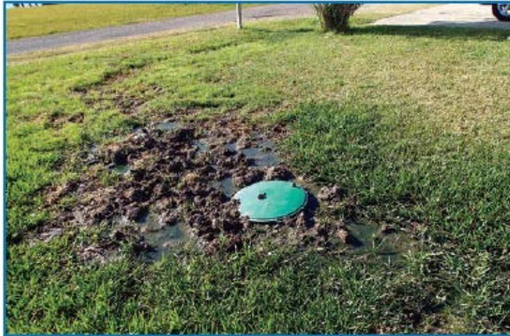
Figure 3: Surfacing of untreated wastewater around a failing OSSF.
